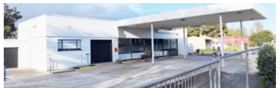
Adelaide Road service station stands abandoned.
