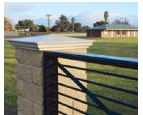
Former netball clubrooms will be demolished at the location of the proposed new office complex on North Terrace.
