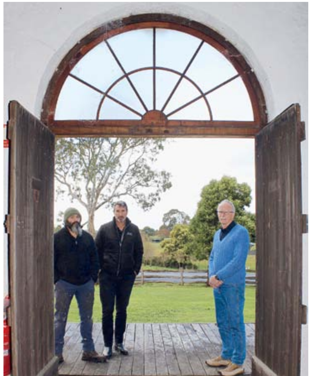
Lighting up: Paul Grima, Peter Allen and Stephen Maxwell stand by the Glencoe Woolshed's arched doorway which still has frosted glass windows waiting for replacement.
