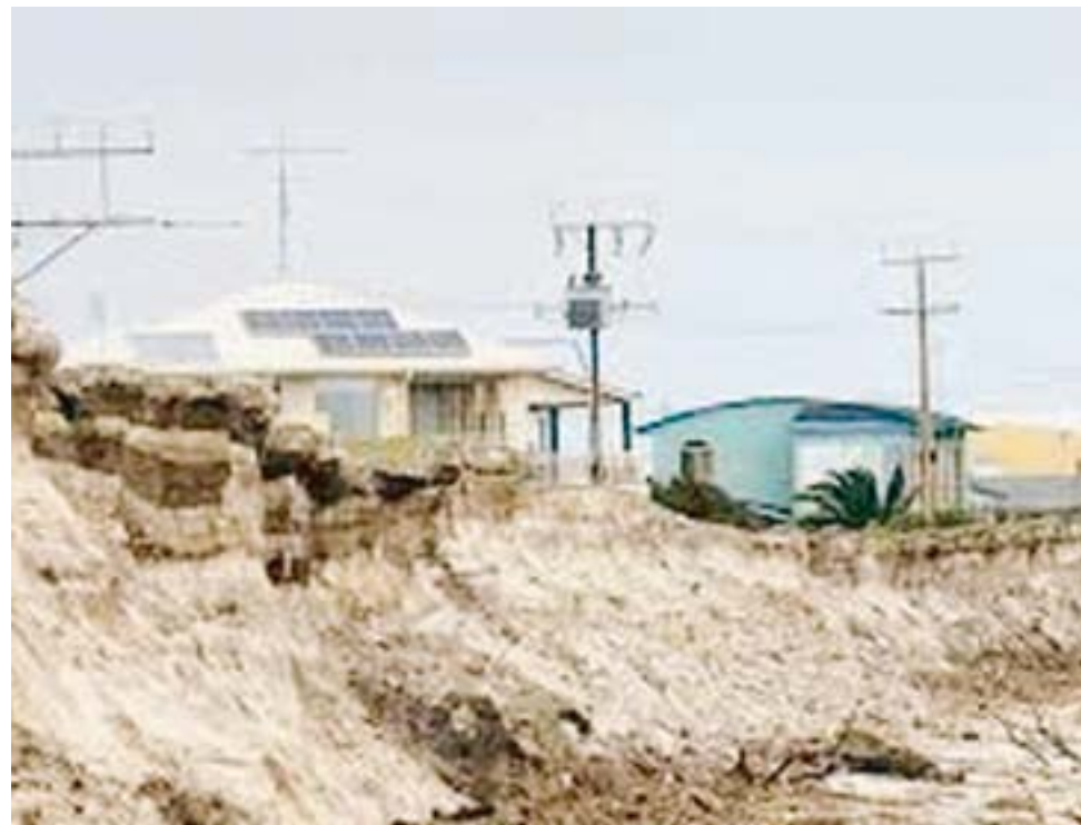
Funding will help to fix erosion issues at Wyomi Beach.
