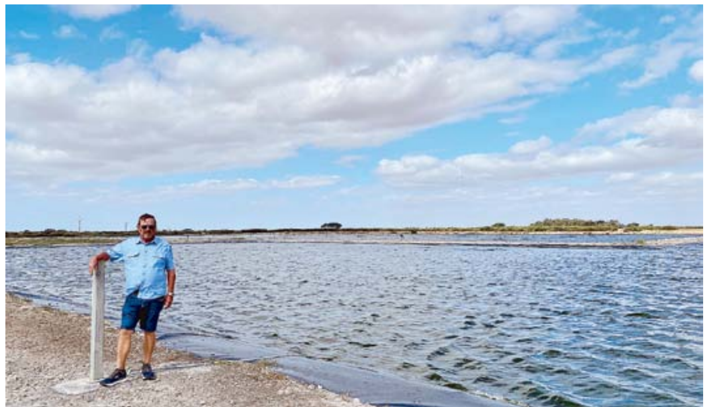
Mayor Jeff Pope pictured at the existing Community Wastewater Management System treatment plant.
