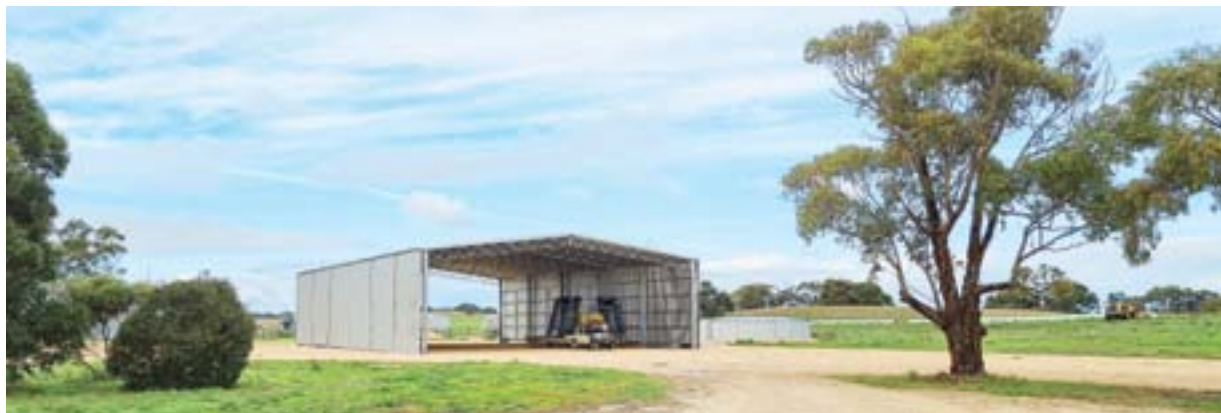
Machinery Shed: A 40m x 24m x 7.5m drive-through machinery shed built by Action at Meningie SA. Visit actionsteel.com.au for inspiration for your machinery shed project.
