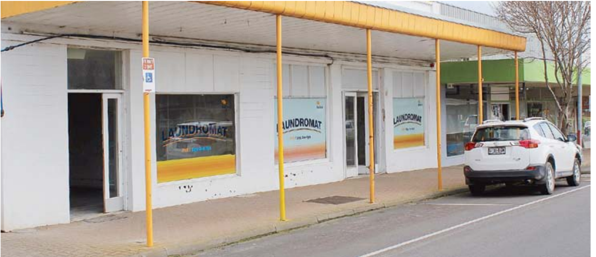
The row of shops which previously housed Bedford Industries is set to become three separate stores.
