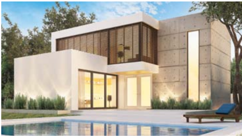
Concrete exteriors are popular exteriors for modern housing. 209918
