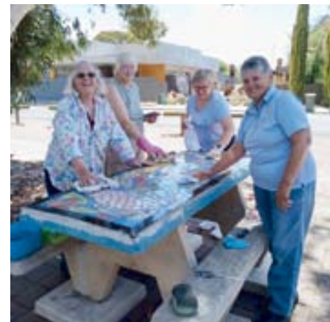
HARD WORK: Val Lewis, Kath Callery, Marcia Camac & Anne-Marie Zanker apply the grout to the the installation.
