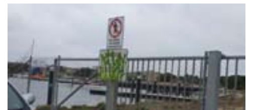
UNSAFE: Some graffiti covered signs meant to warn people of dangerous equipment and areas.
